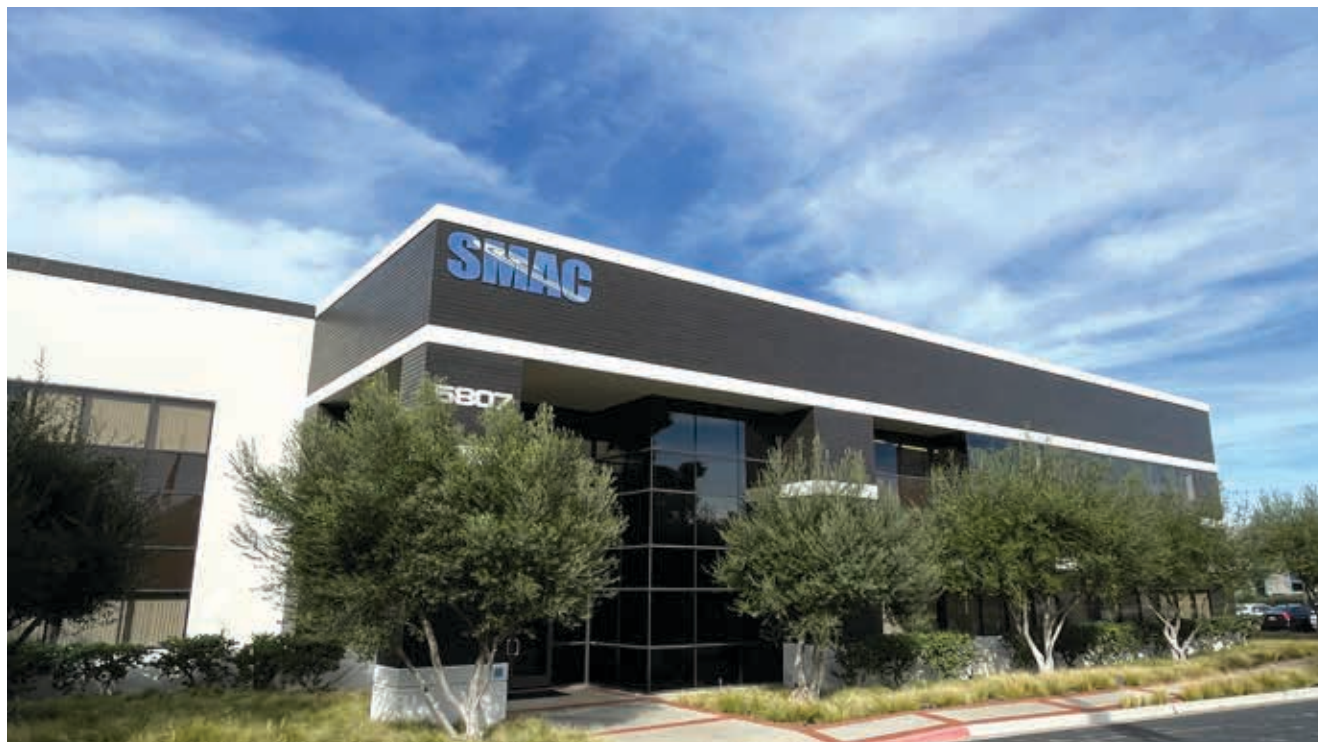
SMAC Corporate Headquarters and Factory
